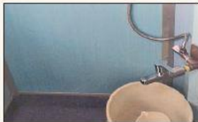
Height of tap raised to accommodate bucket; hand showers provided
