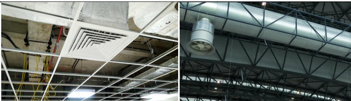
Exposed Metal Ducts
